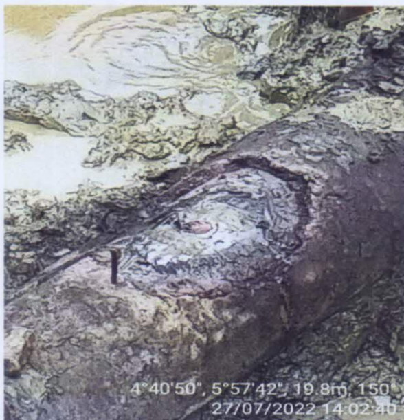
Fig C: Incident facility during repair
